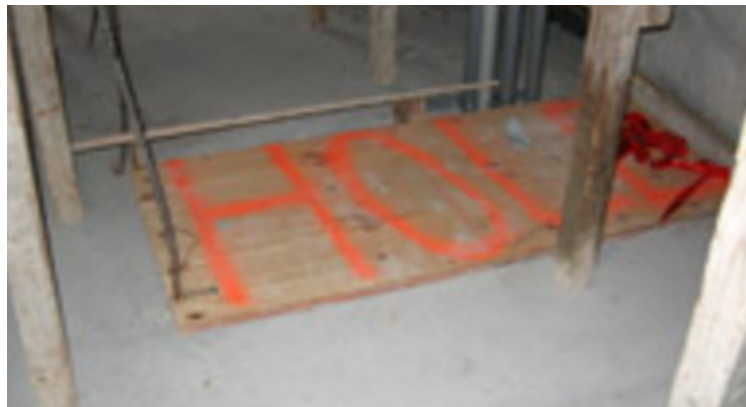
Floor hole cover- Marked hole
