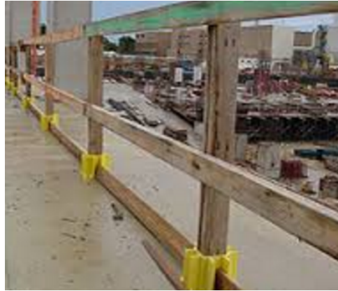
Wooden Guardrail
