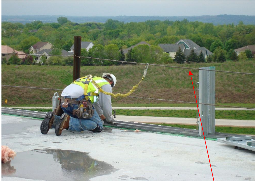
Perimeter guardrail system with engineered fall protection for top rail, missing flagging every six feet
