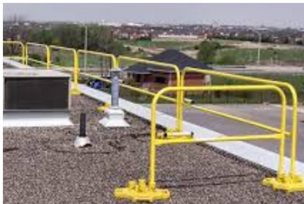
Floor perimeter guardrail system
