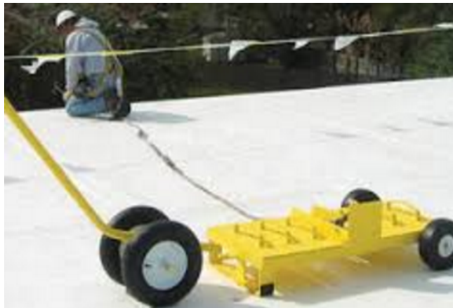
Roof cart anchorage system
