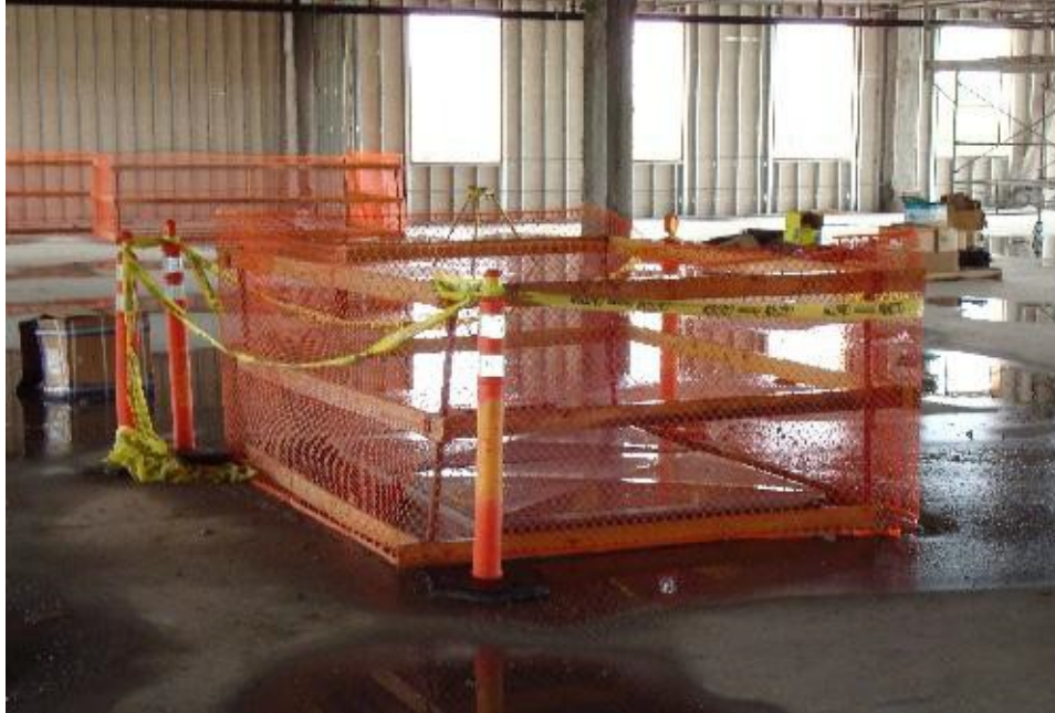
Floor opening with Guardrails and mesh
