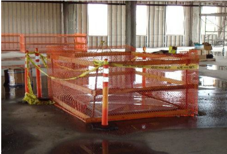
Floor opening with Guardrails and mesh
