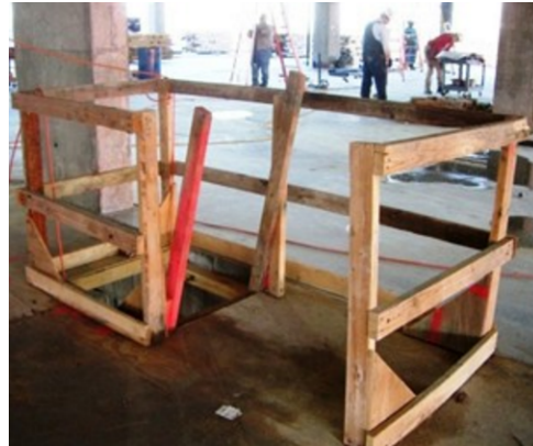
Guarded access point to a roof – fully guarded
