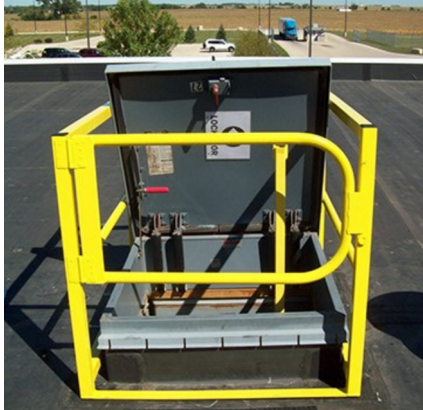
Guarded access point to a roof – fully guarded
