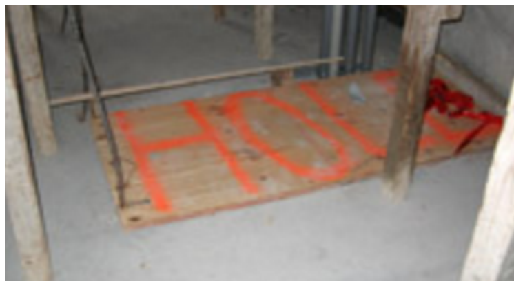
Floor hole cover- Marked hole
