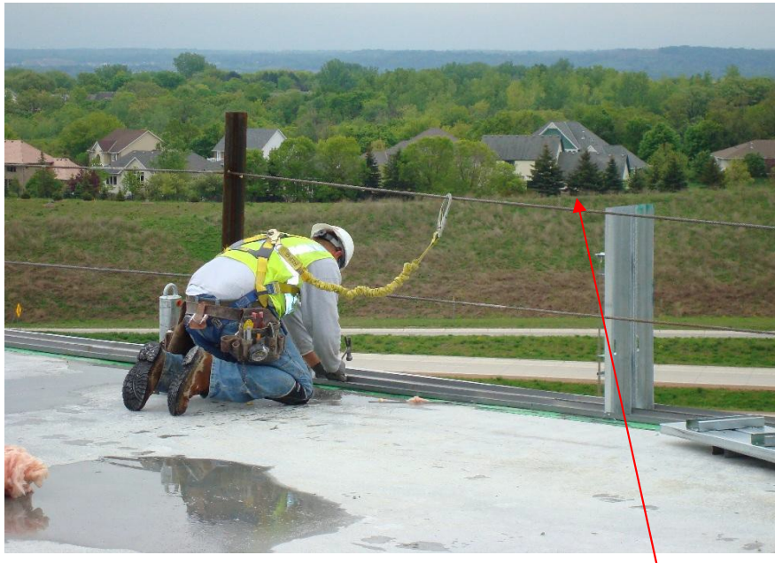
Perimeter guardrail system with engineered fall protection for top rail, missing flagging every six feet
