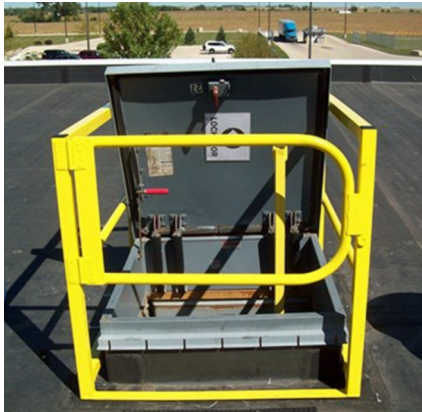
Guarded access point to a roof – fully guarded
