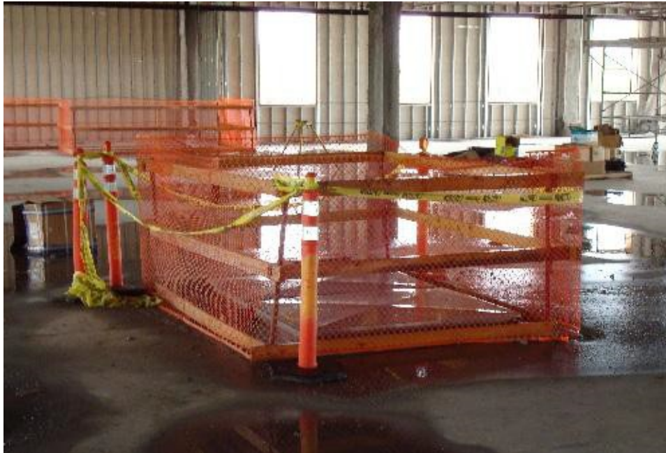
Floor opening with Guardrails and mesh
