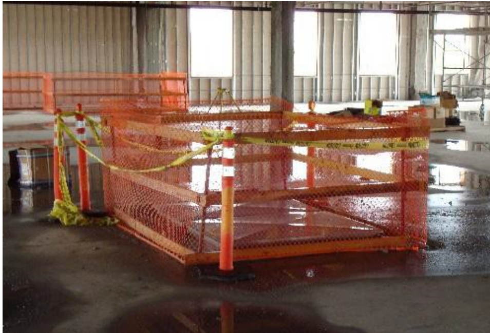
Floor opening with Guardrails and mesh
