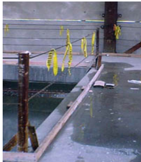
Perimeter wire rope guardrail and toe board with flagging every 6'
