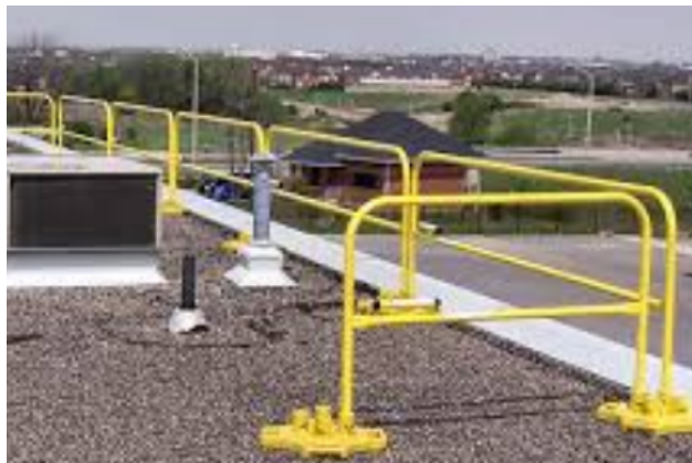
Floor perimeter guardrail system
