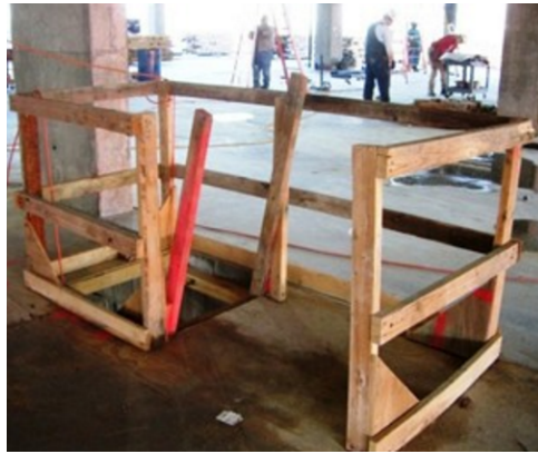
Guarded access point to a roof – fully guarded
